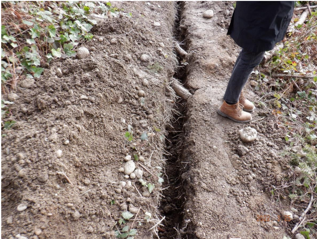
Trench air-excavated south of #23 at proposed cut in grade
